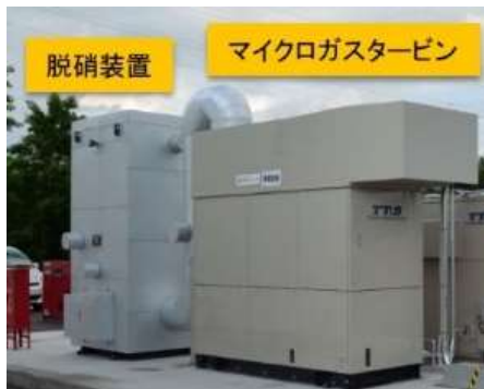
50kW (100% \text{NH}_3 ) Micro Gas Turbine
