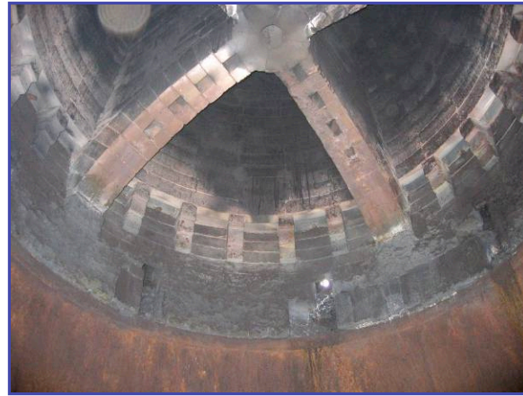
Refractory after 10+ years of operation
