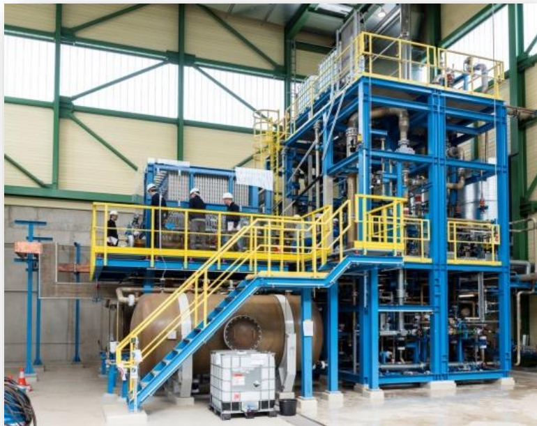
2 MW water electrolysis
