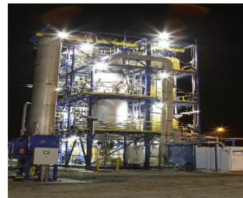
Demo Plant - California
