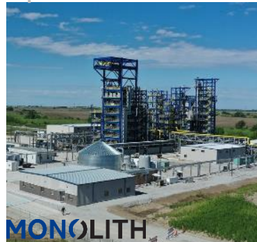
Olive Creek I (OC1), Nebraska Commissioned: 2020
