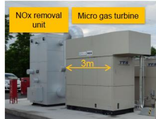
\text{NH}_3 -kerosene-air micro gas turbine in our institute (AIST)
