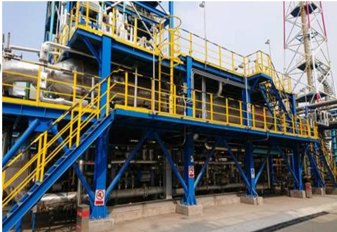
**Measured NO<sub>x</sub>: 50-80 ppm [v] (3% O<sub>2</sub> dry), without “DeNOx”**
